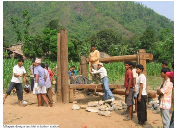
Villagers doing a test trial at bottom station
