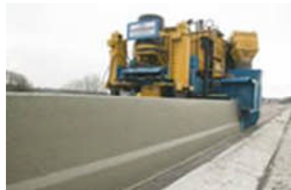
A Slipform Paver in operation
