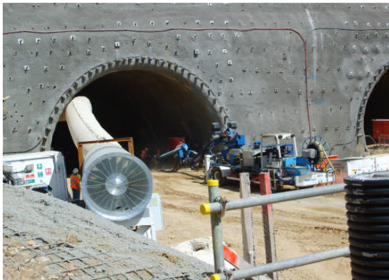
Work at the South Portal – Northbound bore
