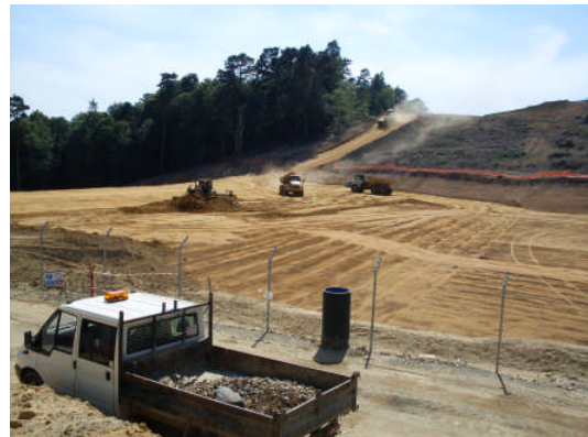
Site levelling on Southern Tunnel Approach
